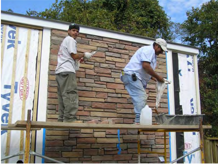
Grouting of the Manufactured Stone
