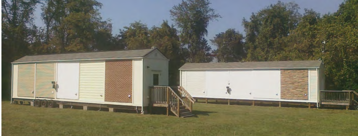
Figure 1: South-facing walls of test structures (building 1 right, building 2 left)
