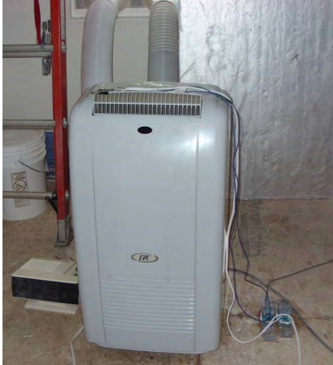
First stage air conditioner with direct vent
