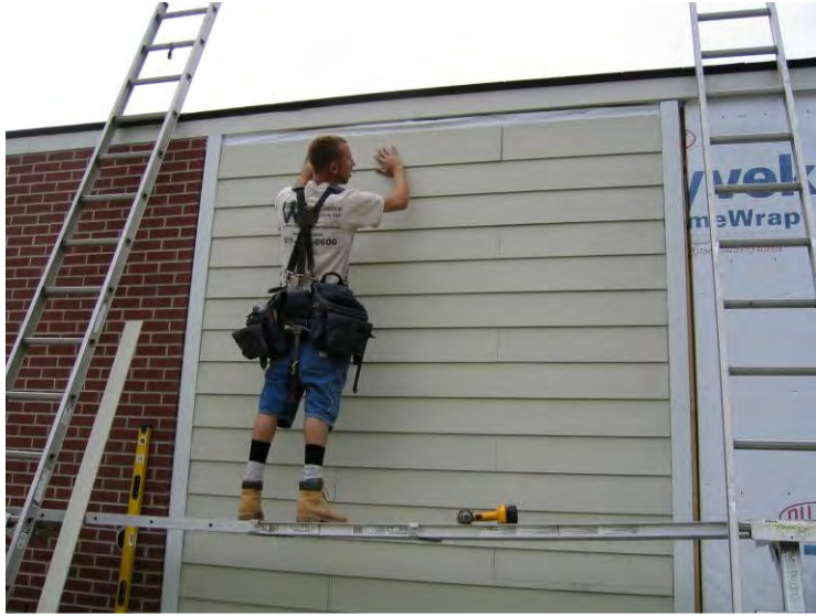
Installing Fiber Cement Siding
