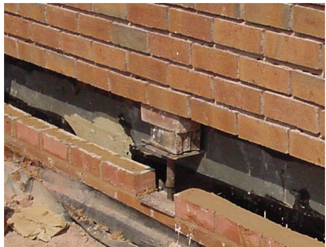
Photo 4 Flashing Installation Using Temporary Support
