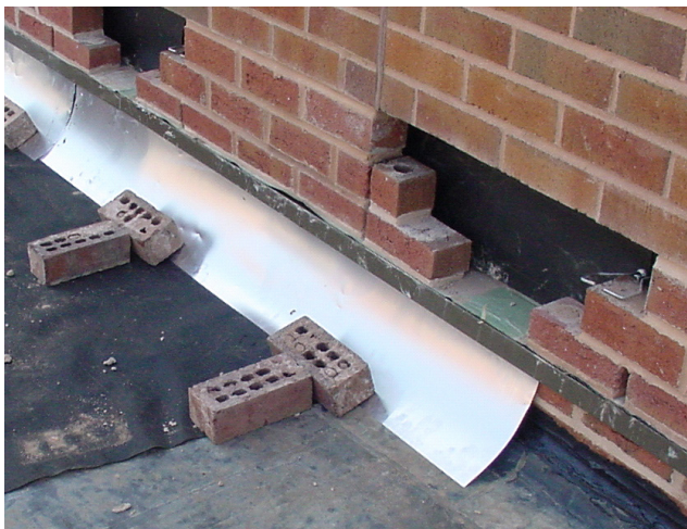
Photo 3 Flashing Installed in Alternating Sections
