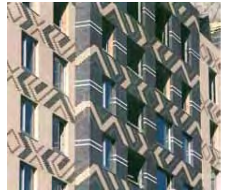
Figure 2. Using brick with different color and texture within brickwork – The Kalahari ©Frederic SCHWARTZ Architects
