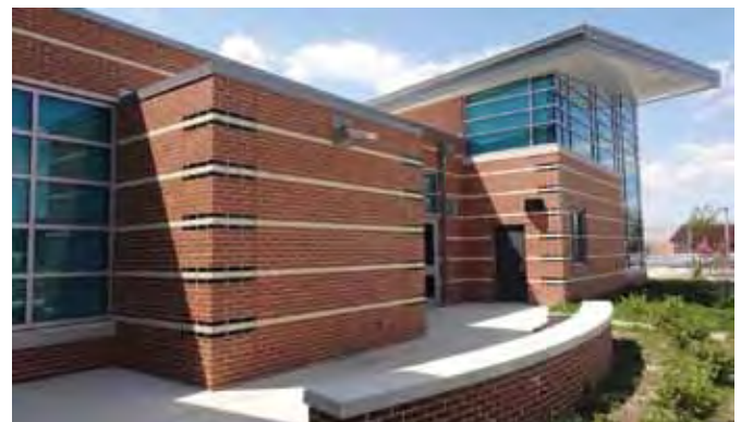
Figure 4. Brick Bands – James M. Bennett High School ©Charles Uniatowski Photography/Becker Morgan Group
