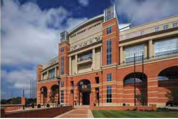
Figure 5. Bands of Other Materials – Deacon Tower ©Jim Sink Photography/Walter Robbs Callahan & Pierce Architects, PA
