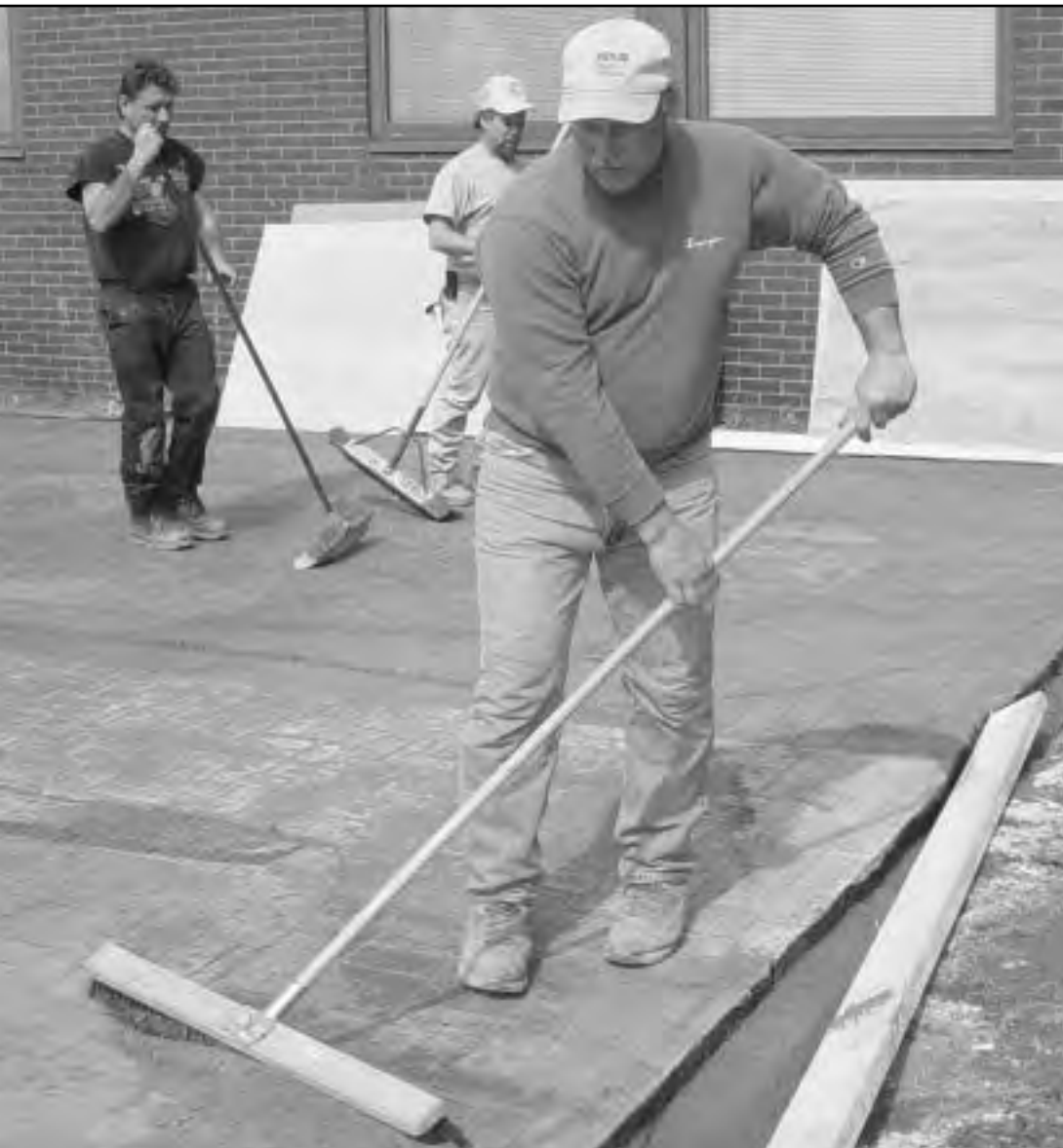
Figure 16: Sweeping Joint Sand
