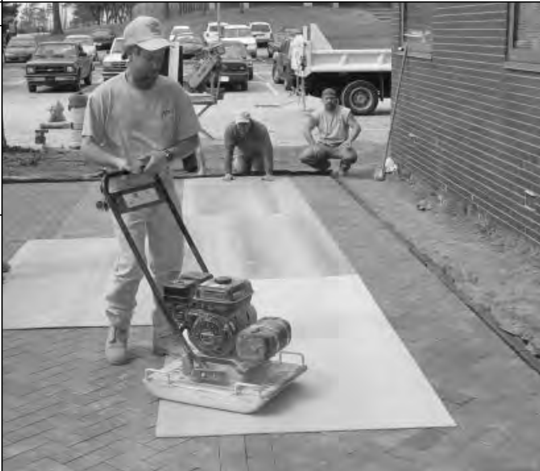
Figure 15: Compaction of Brick Pavers, with Protection
