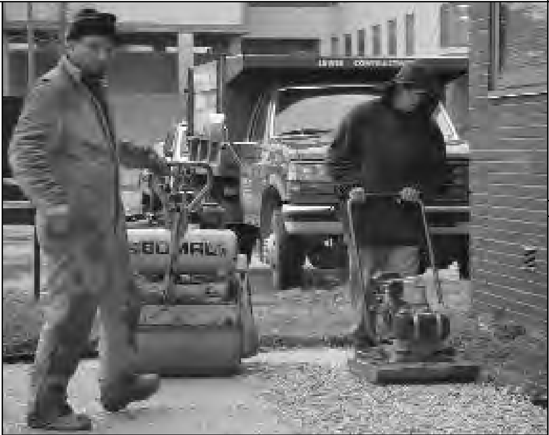
Figure 12: Compacting Near Edge
