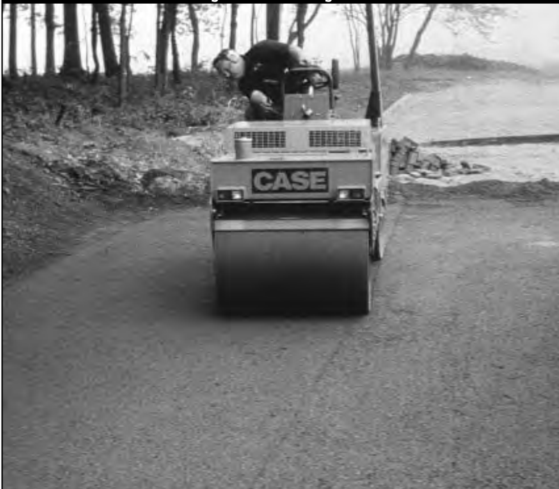
Figure 11: Proper Base Compaction
