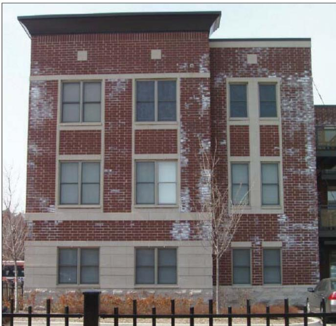
**Photo 1: New Building Bloom.** This type of efflorescence may begin before construction is completed.
