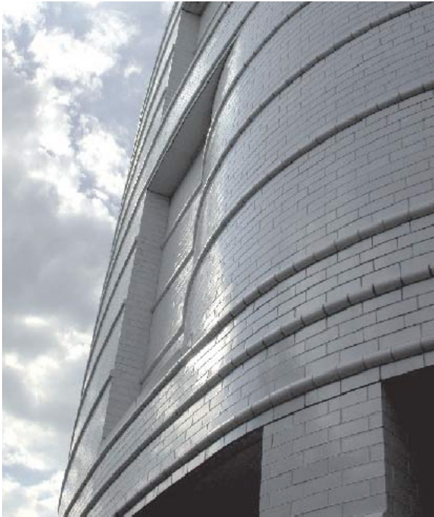
Photo 2 Glazed Brick Used for Entire Facade
