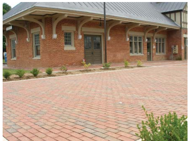
Photo courtesy Pine Hall Brick Company, Inc.
