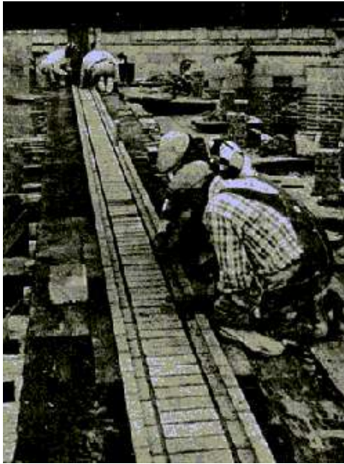
Soffit Brick in Place on Scaffold
