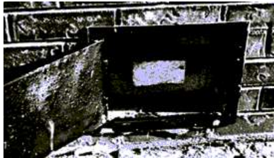
Clean-Out Door Backed with Firebrick
