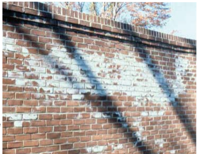
Photo 1 Efflorescence
