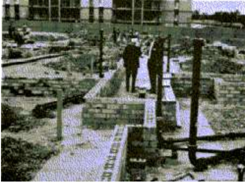
Corridor Bearing Walls at Oakcrest Towers.
