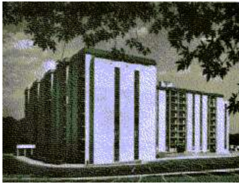
Woodlake Towers, Fairfax County, Virginia
