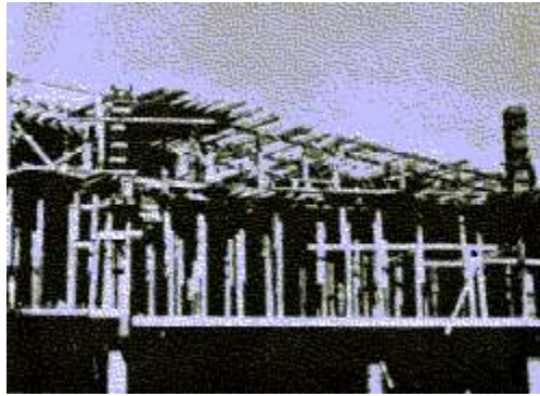
Formwork for Cast-in-Place Concrete Frame.
