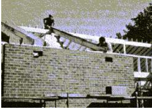
Passive Solar Building with Thermal Storage Wall Under Construction
