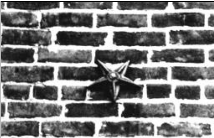
Decorative Through Bolt Bearing Plate FIG. 6
