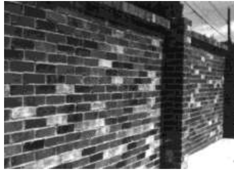
Steel Pier and Panel Wall with Brick Surround FIG. 15
