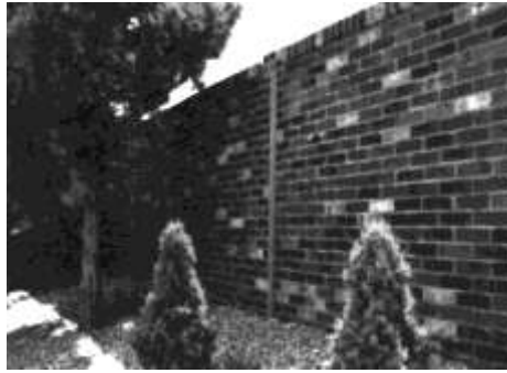
Steel Pier and Panel Wall FIG. 14
