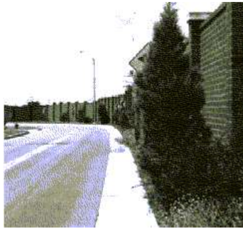
Brick Noise Barrier Wall FIG. 4
