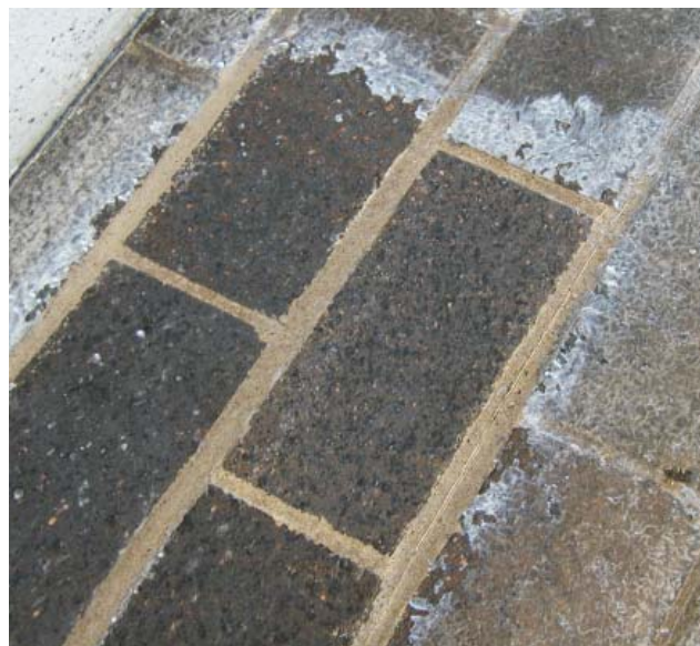
Photo 4 Clouding of a Colorless Coating on a Brick Pavement
