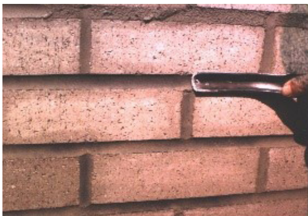
Photo 4 Concave Mortar Joints
