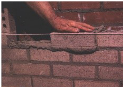
Photo 1 Shoving Brick into Place
