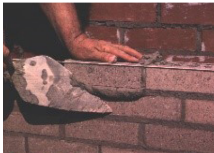
Photo 2 Cutting Excess Mortar
