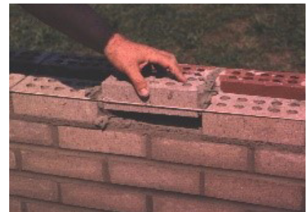
Photo 3 Placing the Closure
