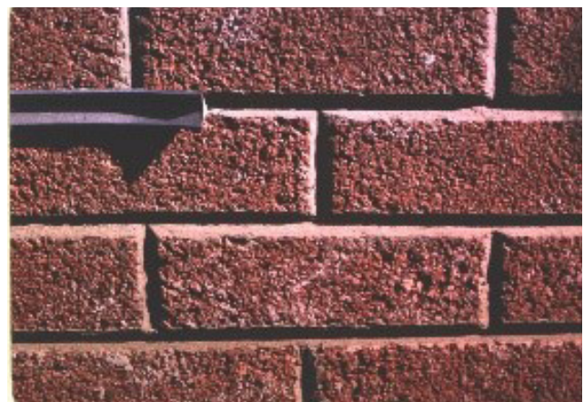
Photo 5 “V” Mortar Joints
