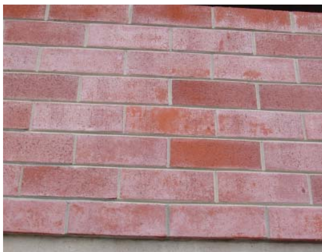
Photo 2 Clouding of Brick Masonry Wall with a Film-Forming Coating
