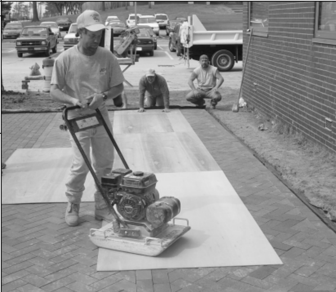
Figure 15: Compaction of Brick Pavers, with Protection
