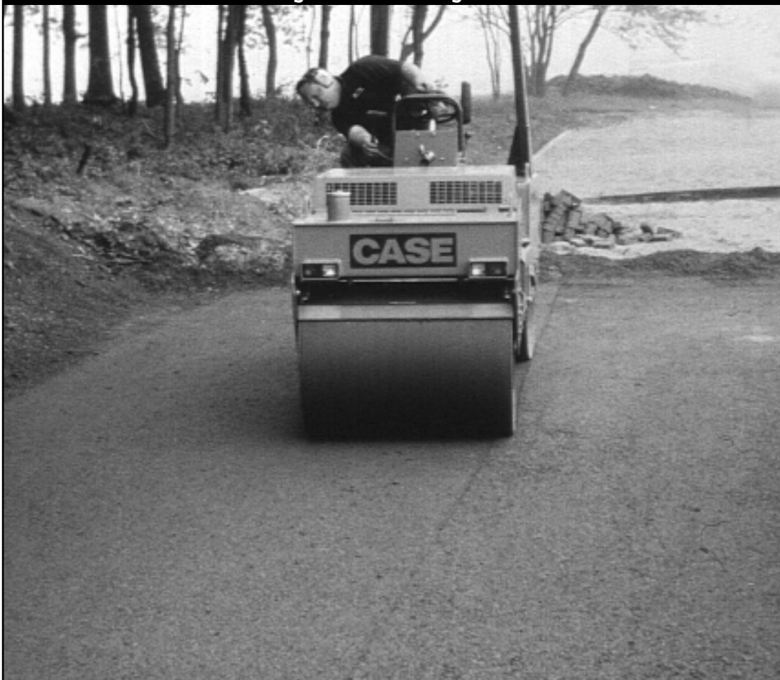
Figure 11: Proper Base Compaction
