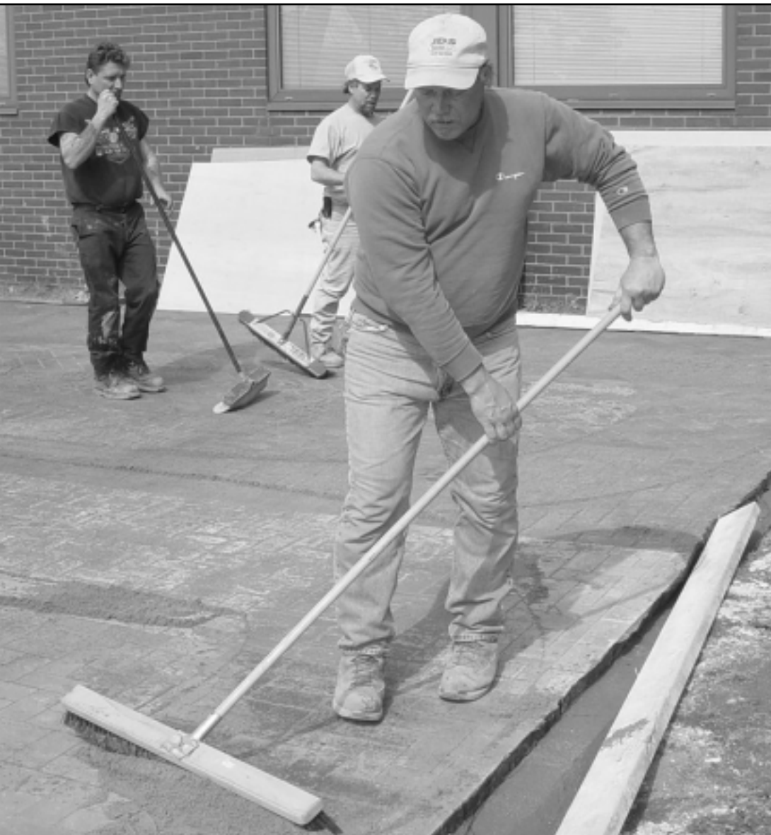
Figure 16: Sweeping Joint Sand
