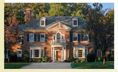
To accurately represent the brick of the Georgian period, the brick was handmade and oversized. Grapevine joints add further complexity to the masonry surface and additional ties to the Georgian tradition of simple elegance. A variety of shaped bricks articulate the home's exterior details, including its water table base, decorative bay panels, corbelled chimney cap, and its straight and round lintels.
