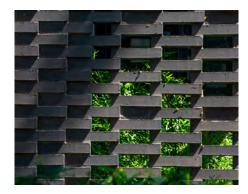
front façade—creates a layer of privacy between the home and the city. The wall's 2-1/4" x 12" solid brick are offset from one another to create a perforation. Carrying the exterior materials indoors allows for seamless spatial flow. Interior brickwork, including accent walls and a large central fireplace, provides eye-catching visual contrast within the bright and airy rooms.
