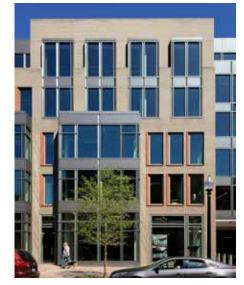
Construction costs met the budget through the use of masonry (vs. curtain wall) and the project's long-term maintenance is significantly reduced due to masonry's weathering properties. By providing 3-inch semi-rigid insulation within a 4-inch cavity behind brick, all of the buildings' wall insulation is outside of the vapor barrier—a significant gain in energy conservation and moisture control—a main functional requirement.
