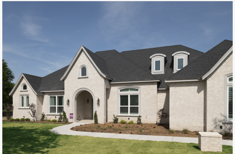
Clay brick exteriors provide a minimum one-hour fire resistance rating.
