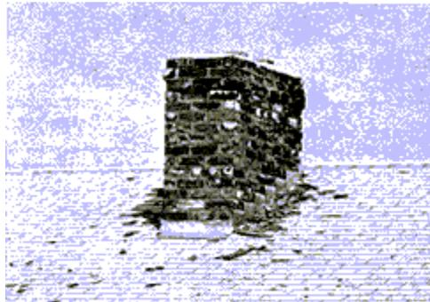
**A chimney of salvaged brick which has spalled considerably within a relatively short time after construction (Knoxville, Tennessee).**
