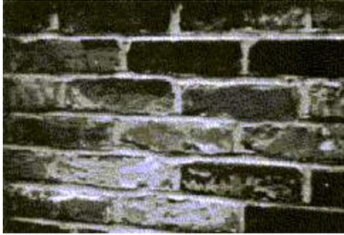
**A close-up of a wall indicating the excessive spalling that is likely to occur where salvaged brick are exposed to weathering.**
