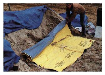
Photo 2 Heating a Sand Pile with an Electric Blanket
