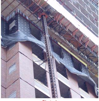
Photo 1 Covering Protecting Newly Constructed Masonry
