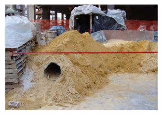
Photo 3 Sand Pile Warmed by Heated Pipe
