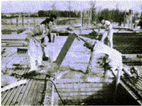
Polyethylene Sheets Under Corridor Formwork in Construction of Oakcrest Towers.
