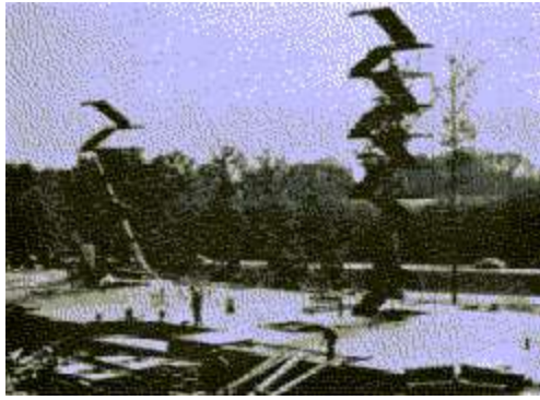
Prefabricated Metal Stairs Used in Bearing Wall Construction.
