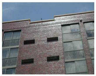
Photo 1 Undesired Gloss Due to a Colorless Coating
