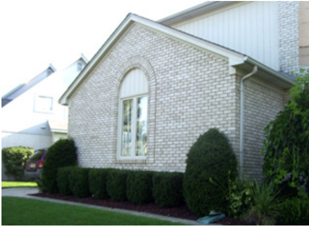
Photo 1 Before Staining Applied
