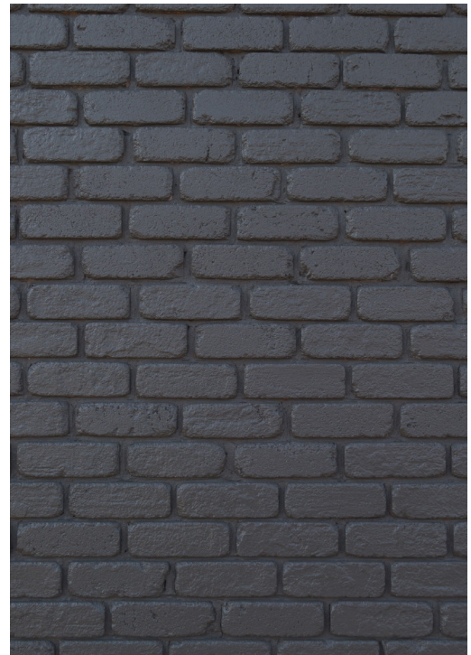
Photo 5 Mineral Paint Finish on Brickwork with Raked Joints
