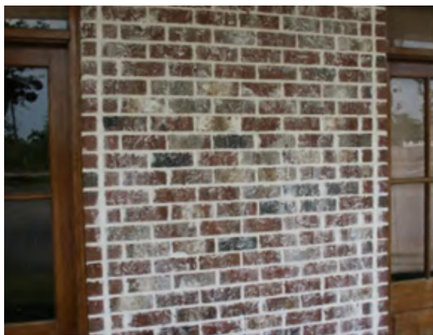
Photo 7 Semi-Opaque Application of Mortar Wash
