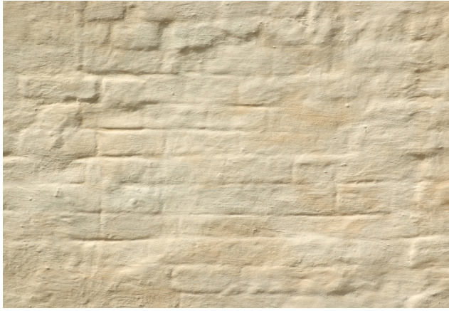
Photo 3 Opaque Finish of Limewash
