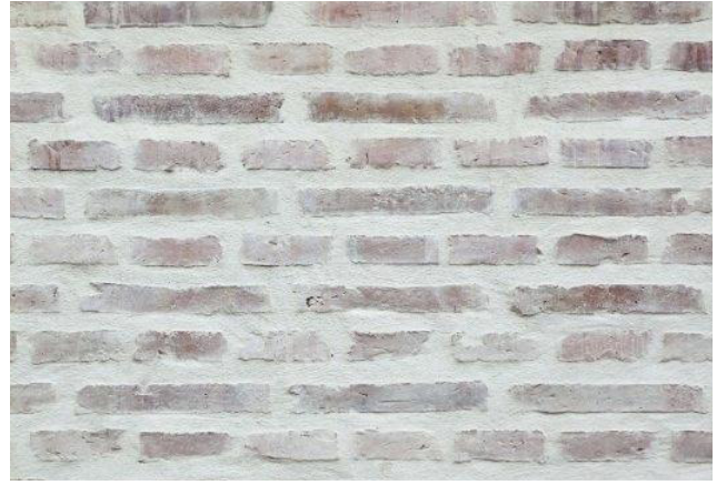
Photo 4 Semi-Opaque Finish of Limewash
