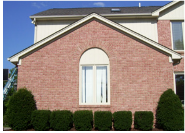
Photo 2 After Staining Applied
